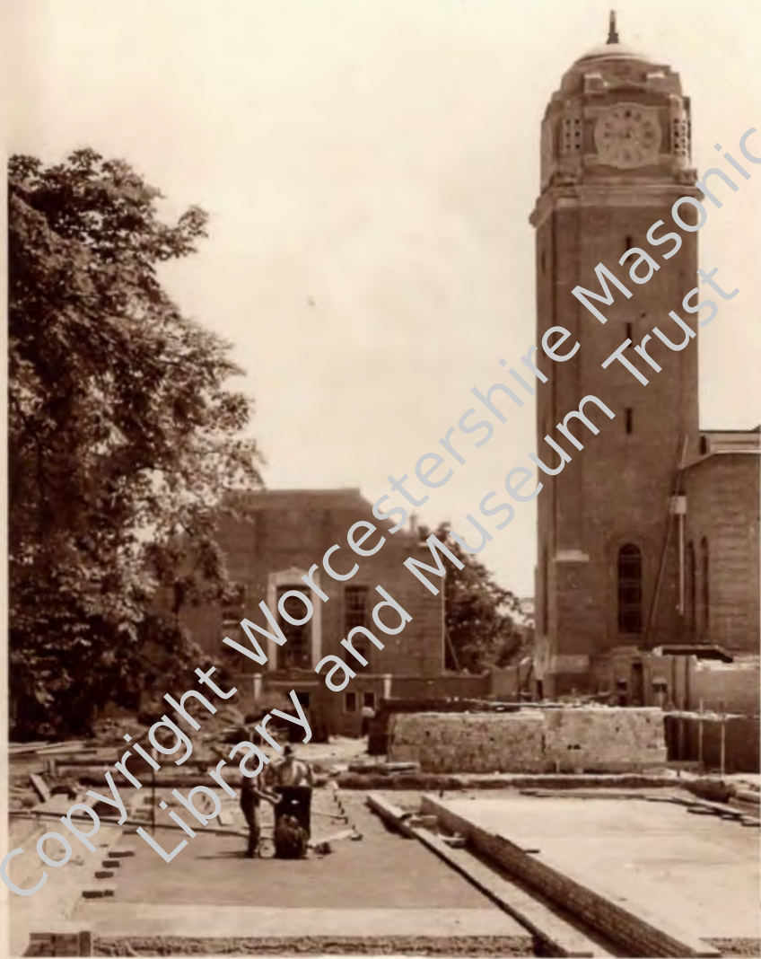
THE TOWER AND THE SITE OF THE CHAPEL: THE DINING HALL IN BACKGROUND
