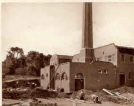
THE BOILER HOUSE. and Central Heating Installation.
